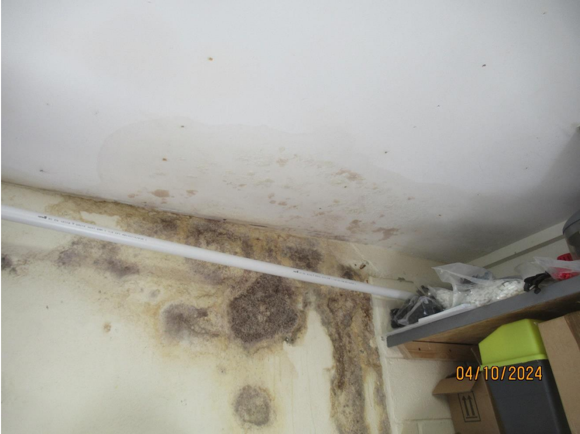
P21 – depot internal concrete wall in store
