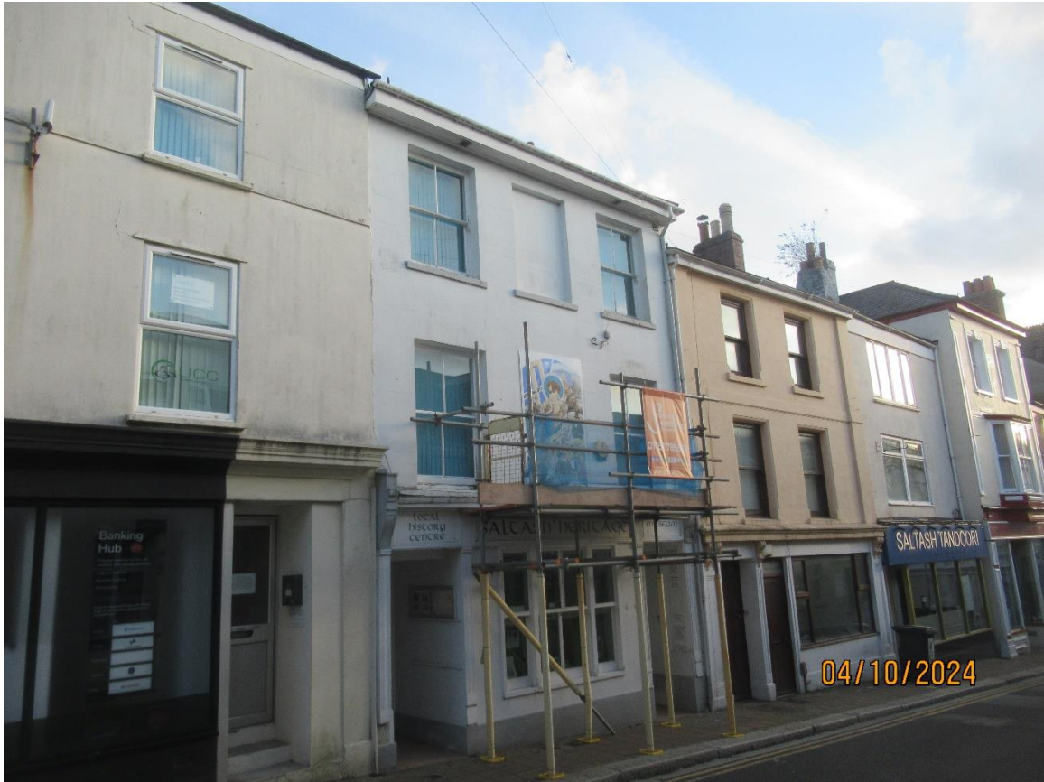
P18 – Heritage building
